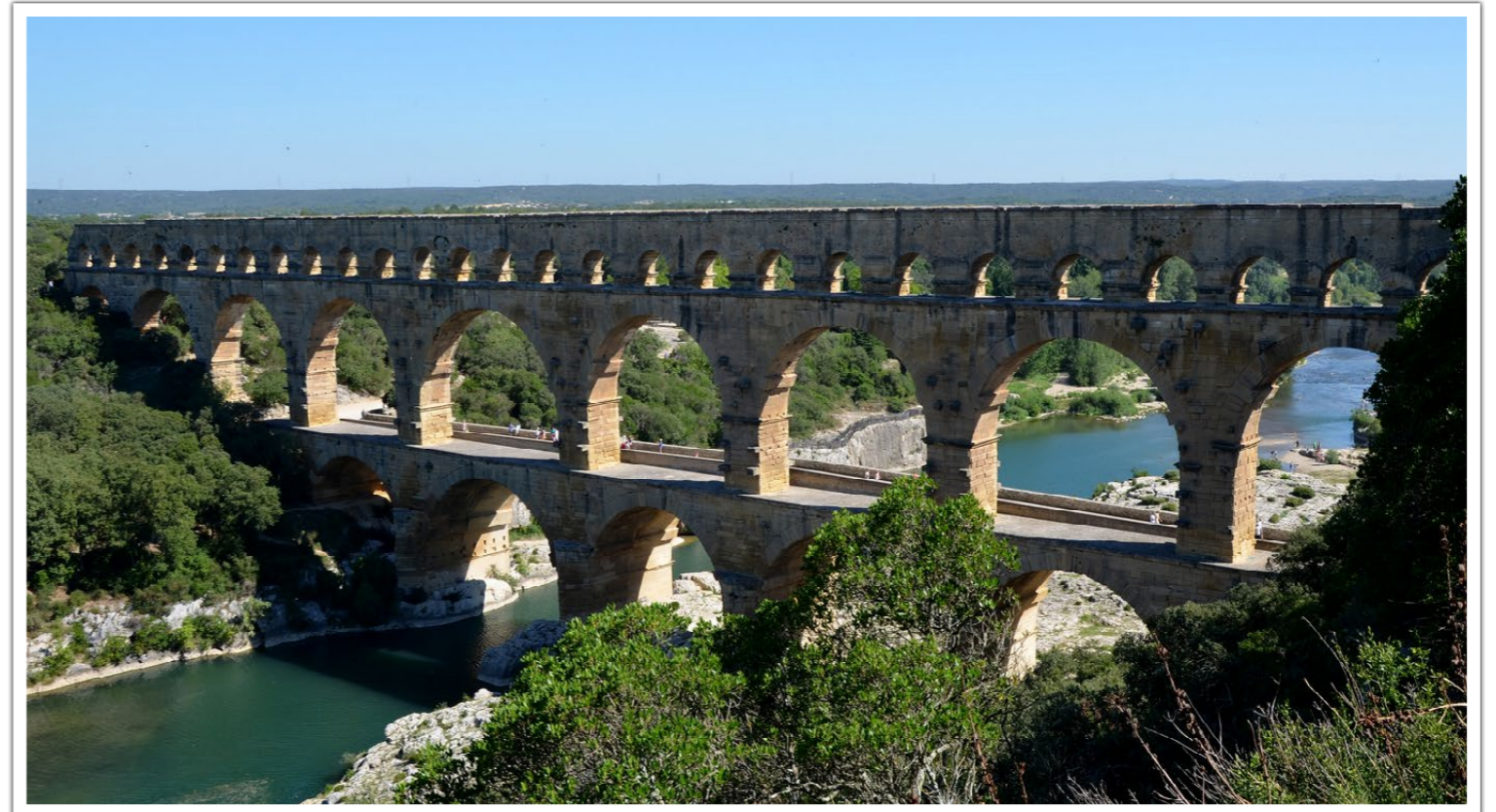
The Pont du Gard located in the Gard at 30 to 45 minutes from St. Rémy
